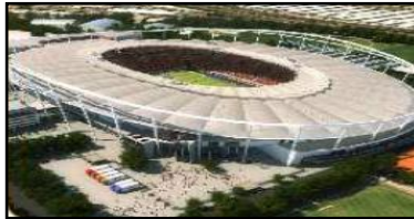
Roof Structure Ropes
