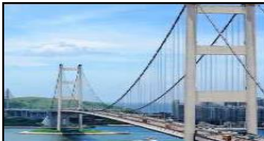
Suspension Bridge Ropes
